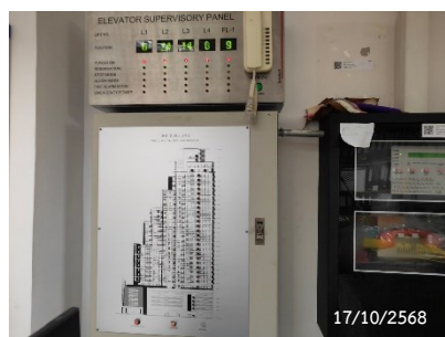
Graphic Annunciator Fire Alarm System
