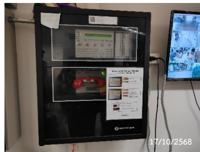
Fire Alarm Control Panel
